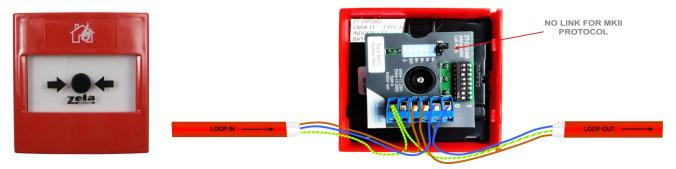
The CP3/AD call point has a built in isolator which can be wired in circuit or not used. This is done by means of not wiring to the negative out terminal on the call point. The following terminals are used for connecting the call point.
