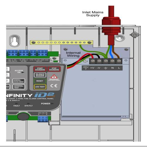
The panel should be connected to 220-240V AC by a 3A rated spur to the fuse box with 1mm<sup>2</sup> to 2.5mm<sup>2</sup> 3-core cable. Nothing else should be connected to this supply. The cable should be fire resistant.
